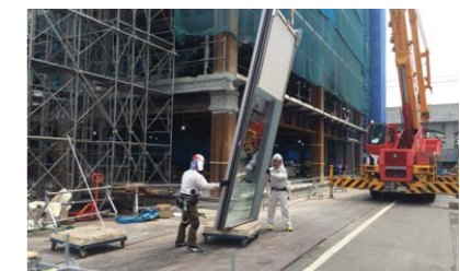
Installation of a unitized CW in progress
