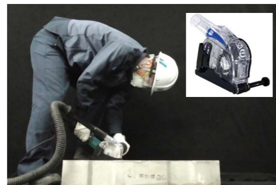
Installation using the "diamond cutter dust collection cover" (top right)
