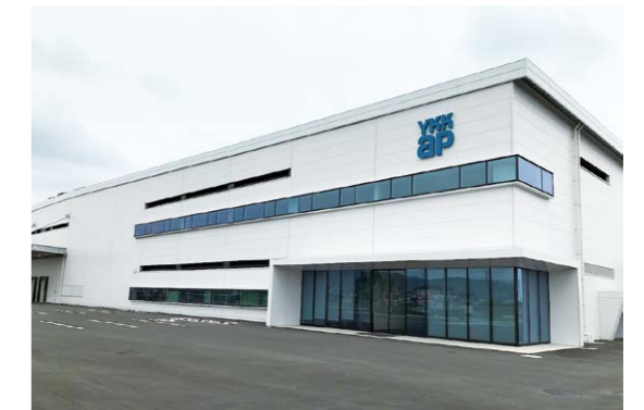
Saitama Factory new building
