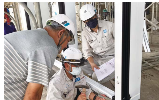
On-site installation training in Taiwan
