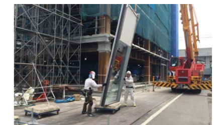
Installation of a unitized CW in progress
