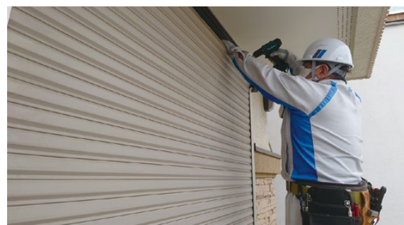
YKK AP Certified Maintenance Technician conducting maintenance on a shutter
