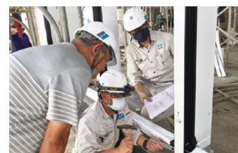
On-site installation training in Taiwan
