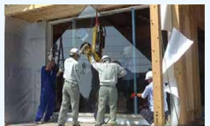
Hoisting Jig for Scaffolding
