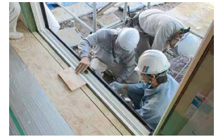
"APW" installation training
