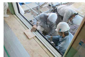
"APW" installation training
