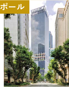
施工例:CapitaSpring Photo: CapitaLand
