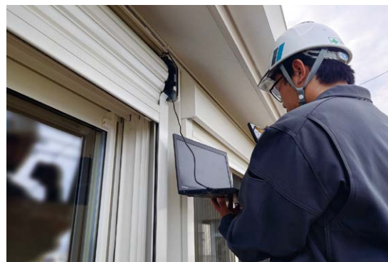
Maintenance of electric equipment using digital tools
