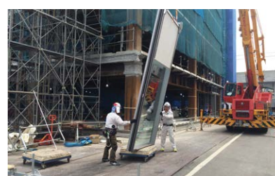
Installation of a unitized CW in progress
