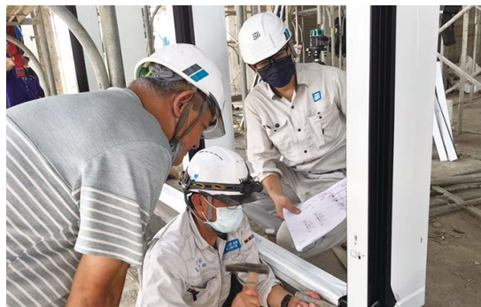
On-site installation training in Taiwan
