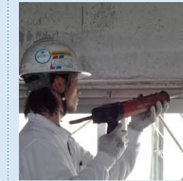
No-weld installation A new flame-free sash installation method that replaces the conventional welding method by filling with mortar.
