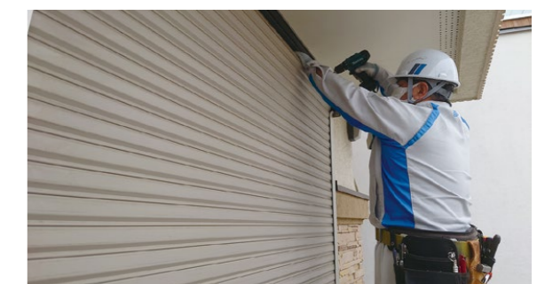
YKK AP Certified Maintenance Technician conducting maintenance on a shutter
