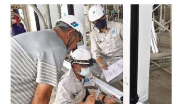
On-site installation training in Taiwan
